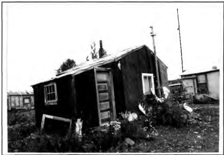
Figure 137. Bunkhouse #1, 1993. The view is looking southeast.
